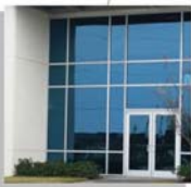
PACIFICA GLASS-BLUE VITRO ARCHITECTURAL GLASS 15% OF FACADE
