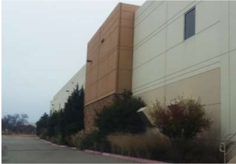
Figure 6-X Landscaping along the base of a façade
