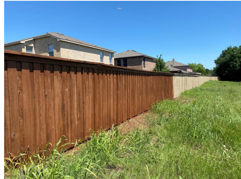
New Fence Stain – Nearing Completion
