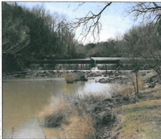
Channel check dam reduces velocities and protects the streambank.
