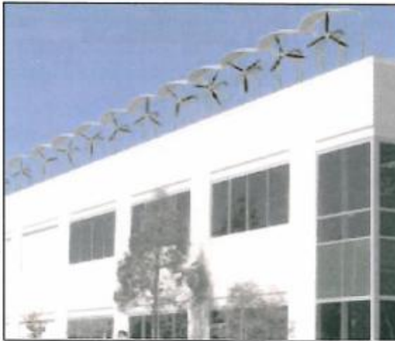
Wind Turbines on a Warehouse (AeroFironment rooftop array).
