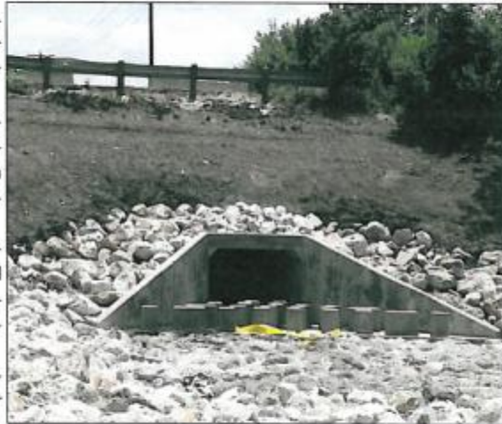
Baffle block dissipates energy on the outflow of a box culvert.
