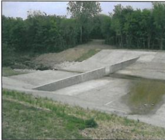
Arbor Creek check dam reduces channel velocities.
