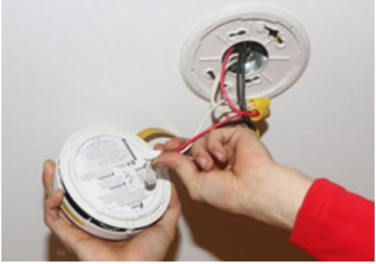
2. Make sure that the breaker to the smoke alarm circuit, or multiple circuits that provide power to the smoke alarms, is turned on.
