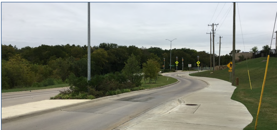
Dechman Drive & Access - looking north
