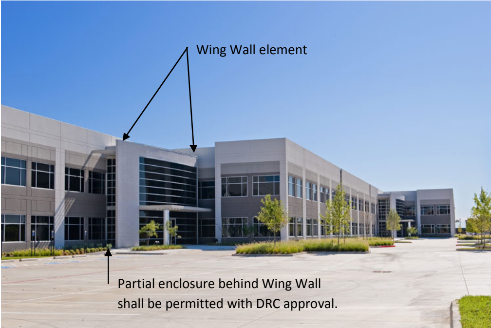
Partially Enclosed Wing Wall Example.
